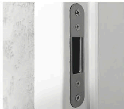
Magnetic lock striker in frame
